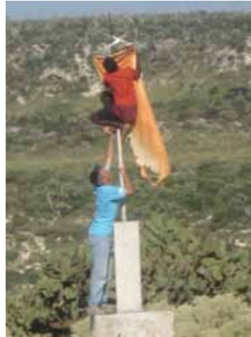
Intergovernmental coordination to repair a windsock
